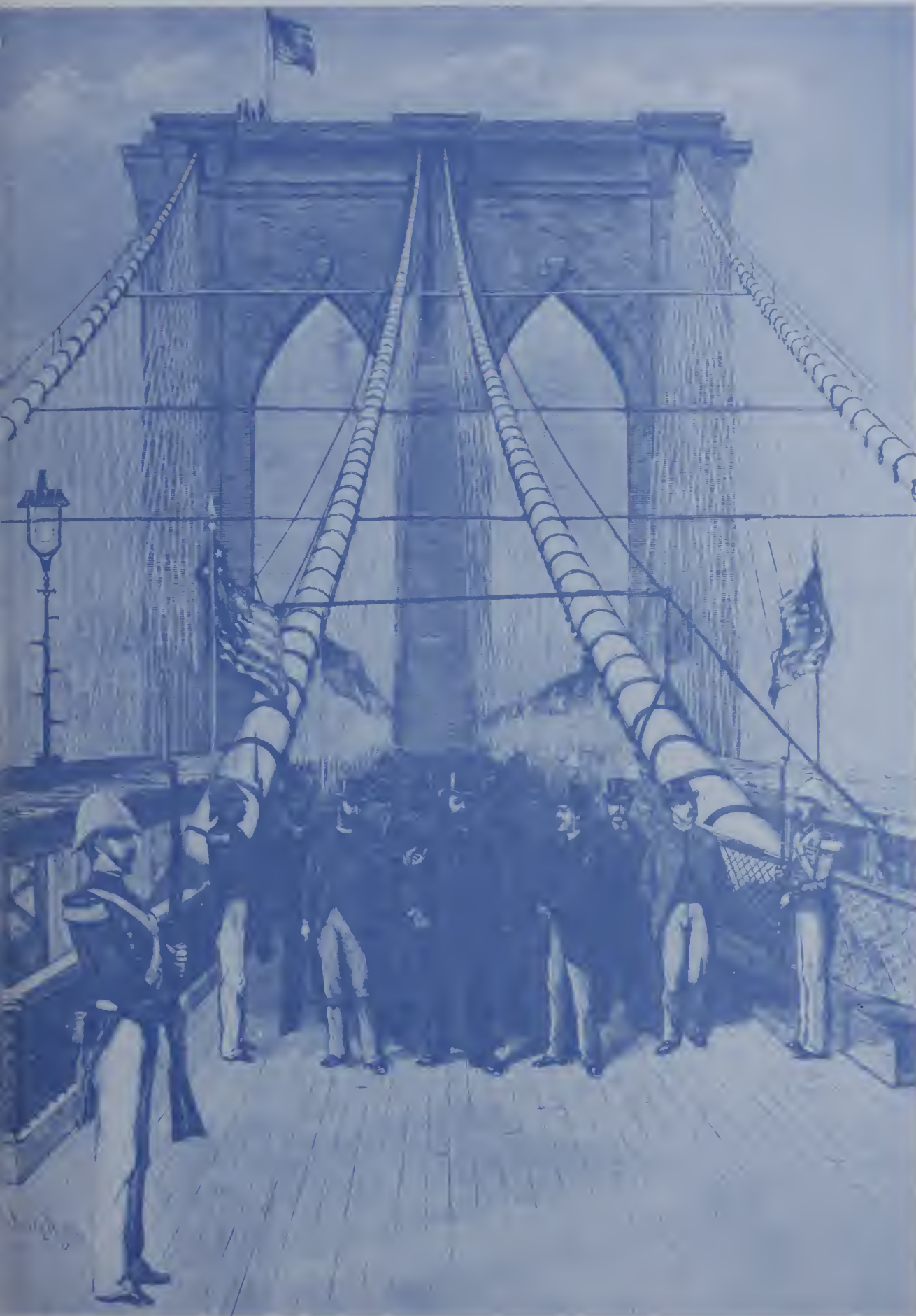
President Chester A. Arthur and his cabinet, Governor Grover Cleveland and his staff, examine the bridge upon opening day, traversing the pedestrian walk.
